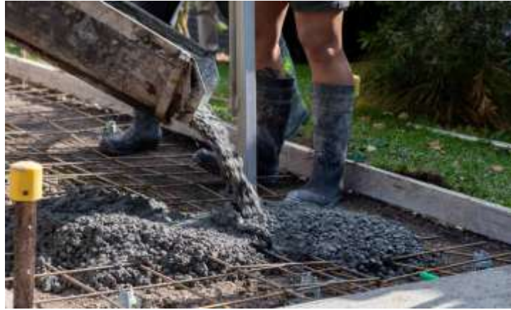
Figure 2. Preparation of coffee-enhanced concrete [URL-1].
