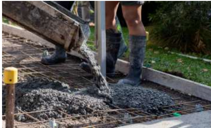
Figure 2. Preparation of coffee-enhanced concrete [URL-1].
